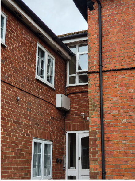
Exterior Structure (The Building)
