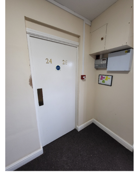
Internal Doors (Compartment Doors)
